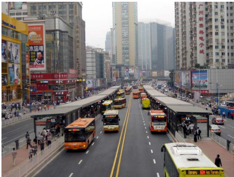
The Guangzhou bus rapid-transit system, before and after. Courtesy Institute for Transportation & Development Policy/Karl Fjellstrom
